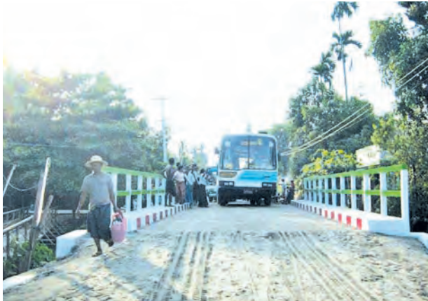
Photo shows newly-built Kyaiklat Pagoda Creek Bridge.
