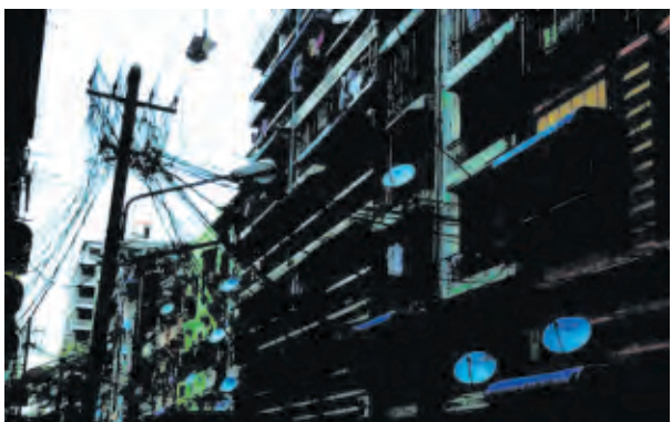
Photo shows electric power lines in a tangle threatening a possible danger of electric fire at the lower block of 43rd street in Botahtaung Township.
