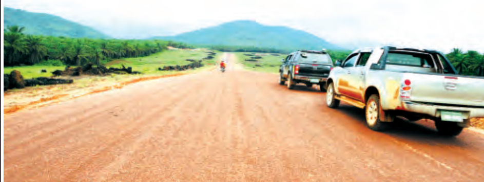
Photo shows Dawei Deep Sea Port section of ASEAN Highway-123.
