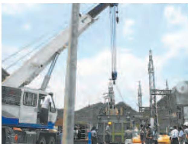
Installation of a new transformer in Lashio power plant in progress.
