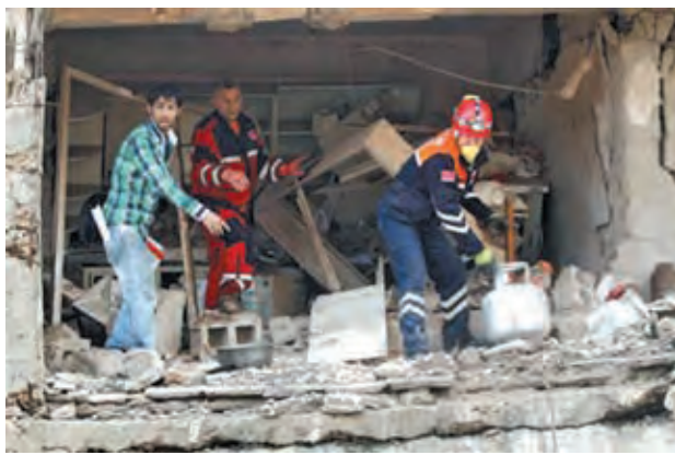
Search and rescue officers work at a damaged building at the site of blast in the town of Reyhanli in Hatay Province, near the Turkish-Syrian border, on 13 May, 2013.—REUTERS
