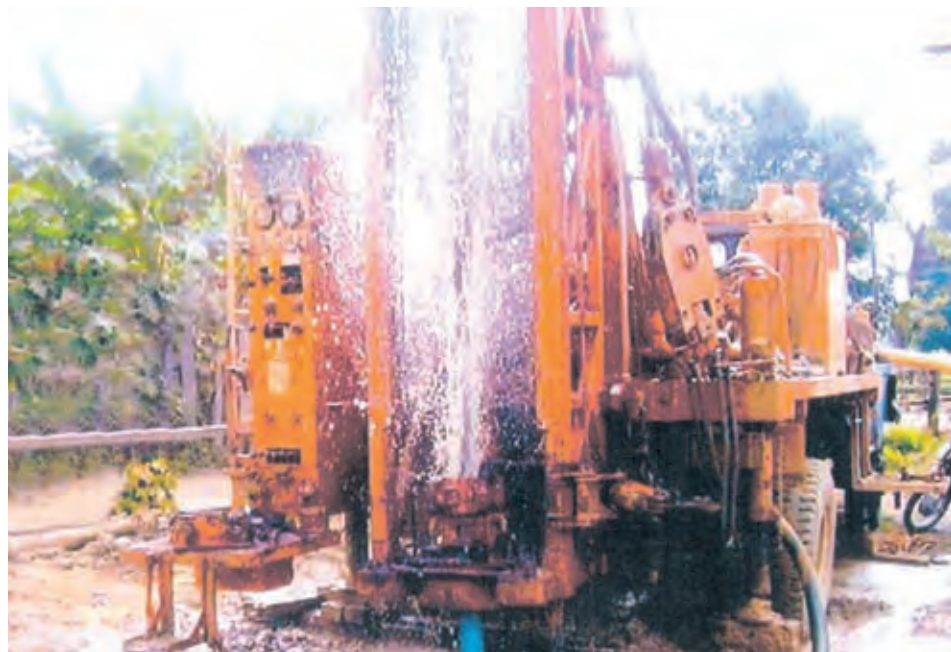
Sinking of tube-well for tapping underground water in progress at dry region.—MNA
