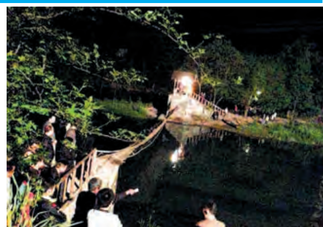
Photo taken on 2 May, 2013 shows the tilted suspension bridge in Fenghuang County, central China’s Hunan Province. About 40 people, who returned from a bonfire party, were on the bridge when the bridge floor suddenly tilted in Fenghuang at around 9:10 pm on 1 May, and more than 20, including children and elderly people, fell into the 1.2-metre-deep river water.—XINHUA
