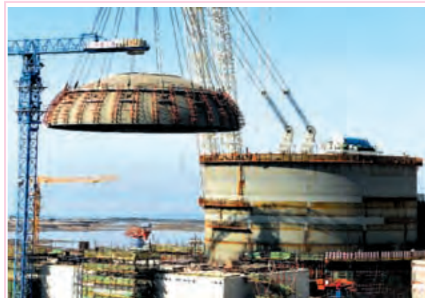
A crane lifts the containment top head to cap the first unit of the Haiyang Nuclear Power Plant in Haiyang, east China's Shandong Province, on 29 March, 2013. The first unit of the Haiyang Nuclear Power Plant, which will be installed with the third generation of nuclear power technology, the AP1000, has seen completion of its civil construction on 29 March. The unit is planned to come into stream at the end of 2014 with annual generation capacity of 17.5 billion Kwh.
