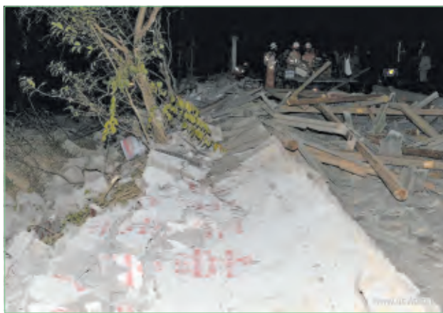
Photo taken on 3 March, 2013 shows collapsed houses after a 5.5-magnitude earthquake in Eryuan County of Dali Bai Autonomous Prefecture, southwest China's Yunnan Province.—XINHUA
