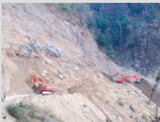
The highway construction passes through steep terrain
