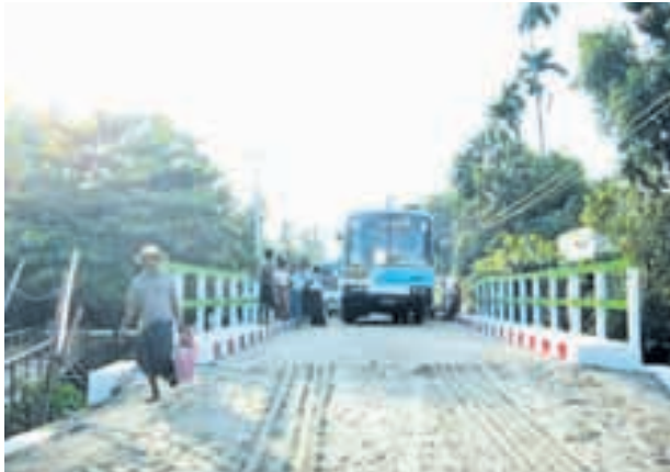
Photo shows newly-built Kyaiklat Pagoda Creek Bridge.
