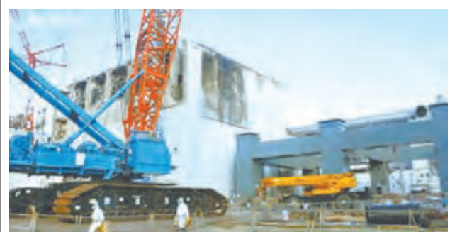
Photo shows the base of a crane facility (R) under construction at the Fukushima Daiichi Nuclear Power Station that will be used to remove spent fuel from the pool of the No 4 reactor building (L) in Fukushima Prefecture on 28 Jan, 2013.—KYODO NEWS
