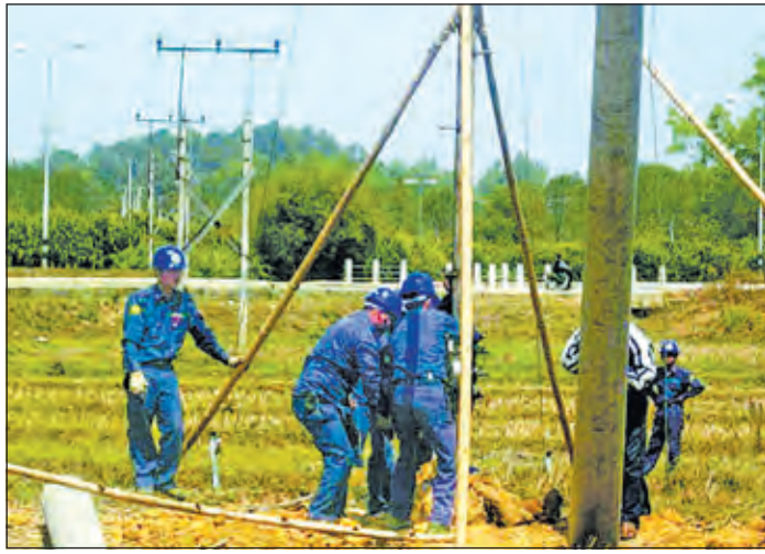
LAMP-POSTS SUBSTITUTED: Skilled workers led by District/Township Electrical Engineer U Han Win Naung substitute old lamp-posts with 10-m concrete posts on 10 January as part of maintenance for 33-kv power grid and safety of electricity in Kengtung of Shan State (East). MYANMA ALINN
