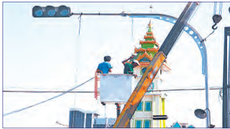
Authority set up the new free line for traffic light between Thanutpin road of Bago and Yangon-Mandalay junction on 11 January. MYANMA ALINN
