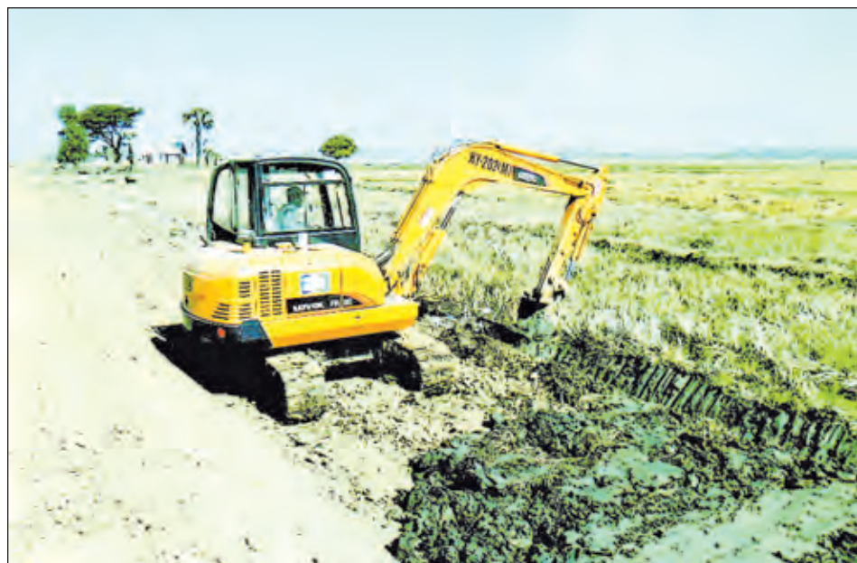
Land reclamation task in progress.
