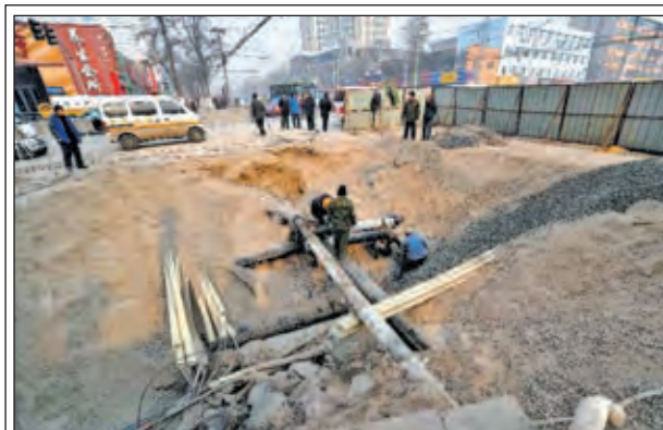
Workers repair the damaged pipelines at the collapsed section of the road intersection of Bingzhou North Road and Bingzhou East Street in Taiyuan, capital of north China's Shanxi Province, on 27 Dec, 2012. The backfilling of the collapsed section has begun, and the damaged pipelines for water and gas supply has been repaired and resumed operation on Thursday, a day after the road cave-in happened. The cave-in left a pit measuring around 3 to 4 meters deep, 15 meters long and 5 meters wide, while damaging pipelines for water, gas and telecommunication.—XINHUA
