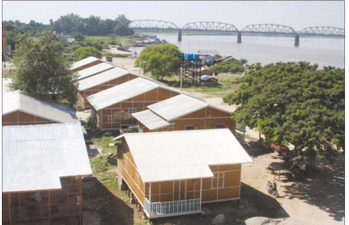
Ministry of Construction houses on land near Yadanarpon Bridge where residents of three villages lived until they were evicted in 2001 for the bridge construction project. Pic: Phyo Wai Kyaw
