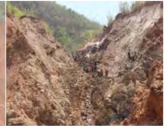
Landslide on 25 April, 2012
