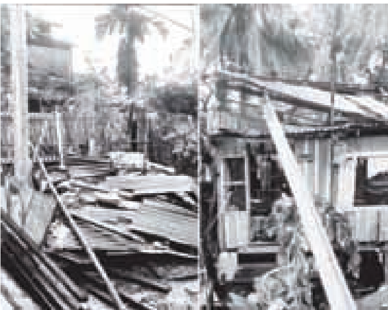
Damages and destroyed houses and property of local people in North Okkalapa Township hit by tornado on 19 July night.
