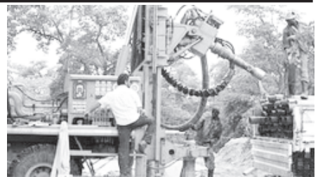
Test drilling on the new aquifer.— INTERNET
