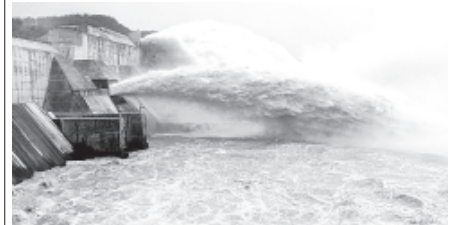
Water gushes out from the Xiaolangdi Reservoir on the Yellow River during a sand-washing operation in Mengjin County, central China's Henan Province, on 20 June, 2012. The Yellow River has been plagued by an increasing amount of mud and sand.—XINHUA
