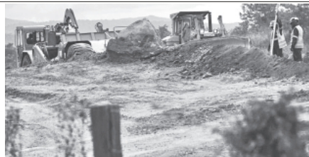
Men work on the expansion of the Carajas Railroad to connect the region of the projected Serra Sul iron ore mine, proposed by Companhia Vale do Rio Doce, to a seaport, in Canaa dos Carajas on 30 May, 2012. Vale is already investing some $11.5 billion in building a port and expanding the railroad line to the region around Serra Sul, as it awaits the mining license which has been held up by the government after archeologically and environmentally sensitive caves were found at the site, Brazilian media reported.—REUTERS
