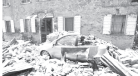
A car is covered in debris after a quake-damaged house collapsed in Cavezzo. A strong earthquake has rocked northeastern Italy, just days after another quake in the same region wrought death and destruction. — REUTERS
