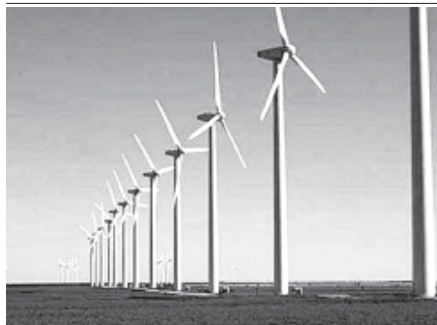
Green Mountain wind farm in Langford, Texas.
