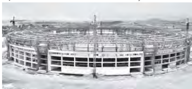
Photo shows progress of Zeyathiri Advanced Stadium.
