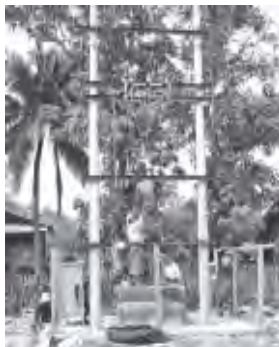
Electricians installing transformer in Mawlu region.
