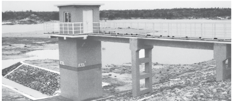
Control Tower of Ngachin Dam.
