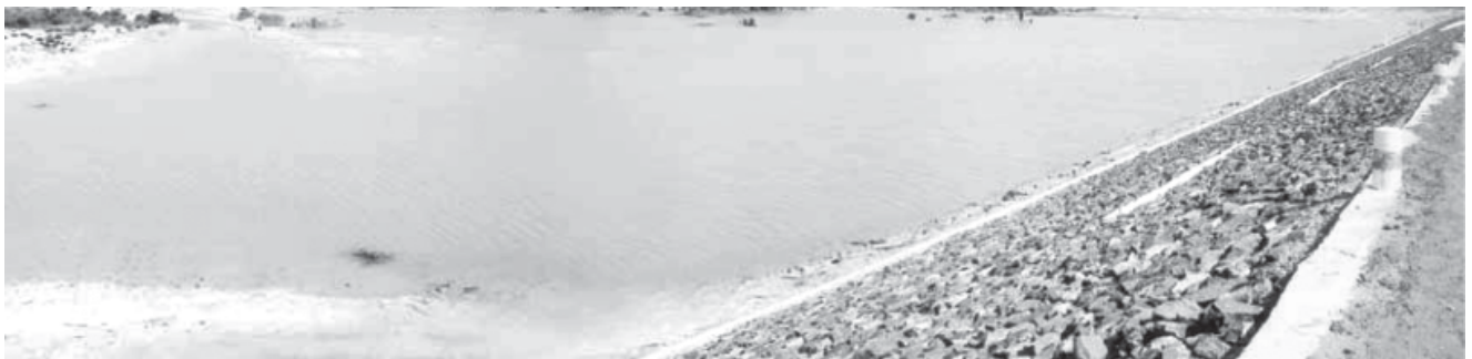
Photo shows Kyauksauk Dam.
