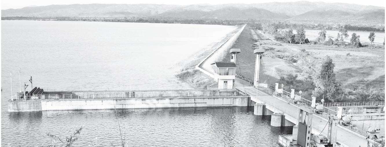
Moby Dam near Moby village in Pekhon Township of Shan State (South) generates electricity and supplies irrigation water.
