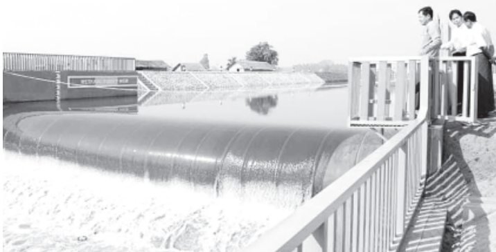
Union Minister for Agriculture and Irrigation U Myint Hlaing inspects Wakkamu Rubber Diversion Weir built through Rubber Dam Technology for the first time in Myanmar on the Nyobin Creek near Wakkamu Village of Lewe Township. —MNA
