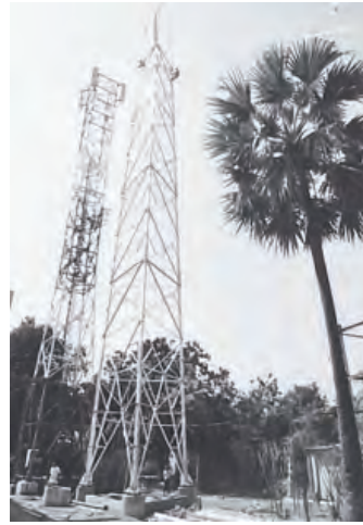
450 metres high communication tower being built by Yatanarpon Teleport at communication station in Yesagyo Township.
