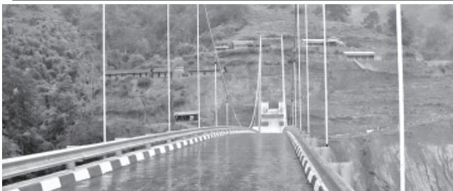
Neat and tidy Thanlwin Bridge (Tarpa).
