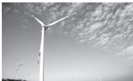
File photo taken on 10 Nov, 2011 shows Laoyemiao Wind Power Plant in Duchang County, east China's Jiangxi Province. China installed 18 gigawatts of wind power turbines in 2011, capturing about 40 percent of the global total and pushing up China's total installed wind power capacity to 62.7 gigawatts, the Global Wind Energy Council (GWEC) said in a report on 7 Feb, 2012.—XINHUA
