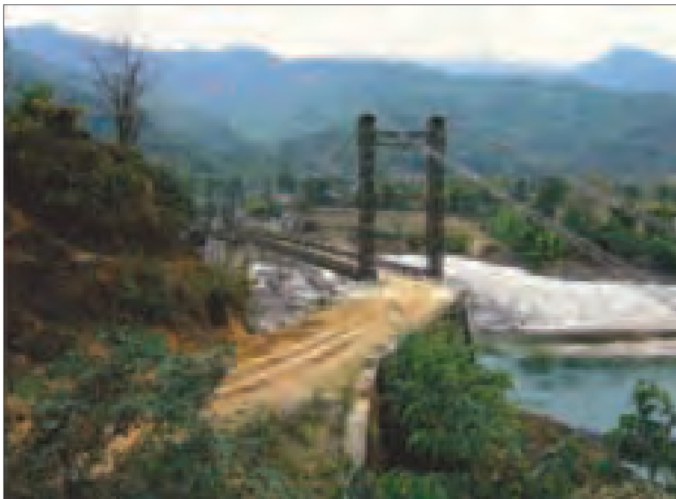
The Chipwe Bridge
