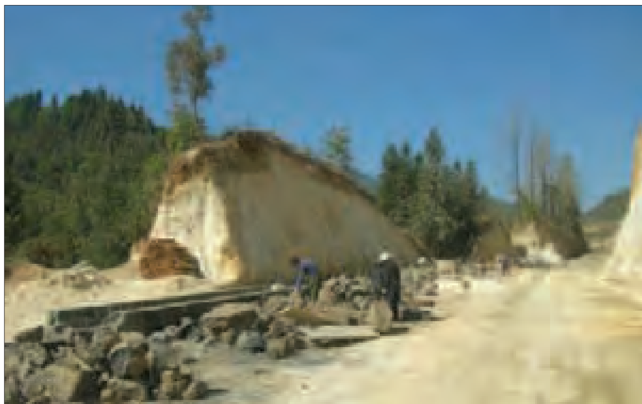
Road building, Guyong; January 2007
