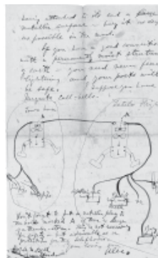
This image released on 5 Jan, 2012, shows a page of an 1878 letter sent to his parents by Alexander Graham Bell. The drawing and accompanying discussion instructs how to ground the telephone Bell had invented. The letter is being auctioned by Amherst, NH, dealer RRAuction. INTERNET
