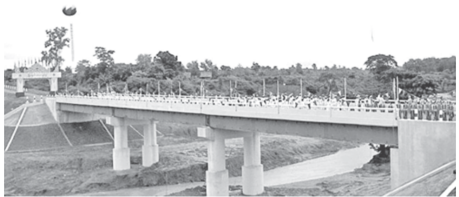
Photo shows already-inaugurated Myo Creek Bridge.
