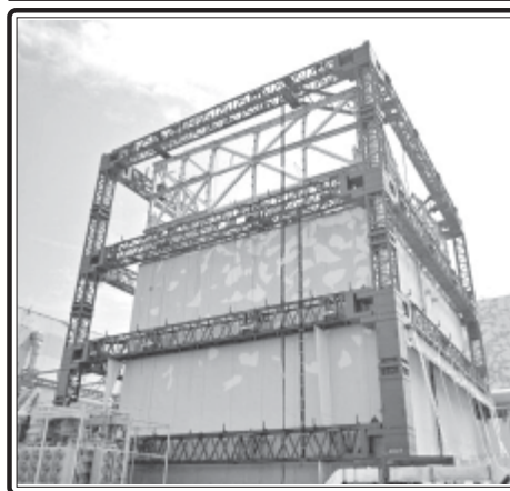
Steel frame constructed for the cover of Tokyo Electric Power Co (TEPCO)'s Fukushima Daiichi Nuclear Power Plant's Unit 1 reactor is completed in this handout photo taken by TEPCO in Fukushima Prefecture, northern Japan, on 9 September, 2011 and released on 10 September, 2011. INTERNET
