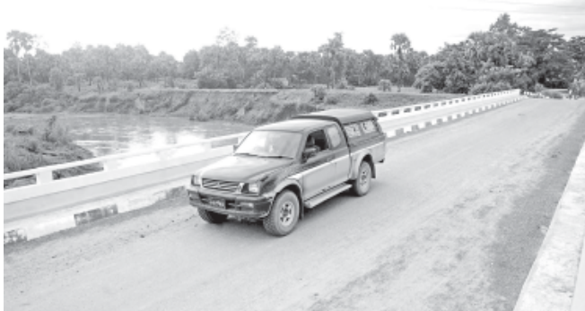
"Vehicles can pass through Ma Mya Creek Bridge."
