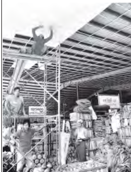
Photo shows ceiling tiles being installed at complex (B) of Thiri Mingala Market.
