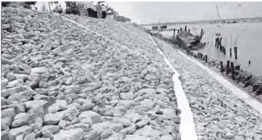
A stone-filled embankment section built by Nyaungdon Township Development Affairs Committee.
