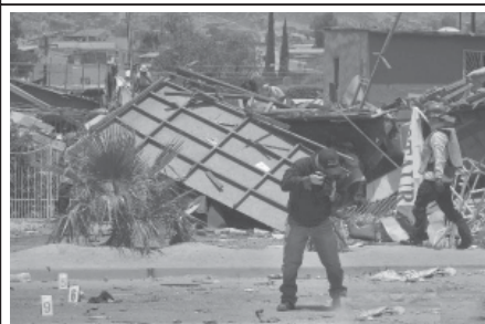
Investigators, firefighters and rescuers work at the blasted Chinese restaurant on the main street of the neighbourhood "El Florido", in Tijuana, Baja California, northern Mexico, on 19 June, 2011. A strong explosion caused by gas leak destroyed the restaurant on Sunday. Twenty six were injured, six of them seriously, sources within the local rescue services informed.
