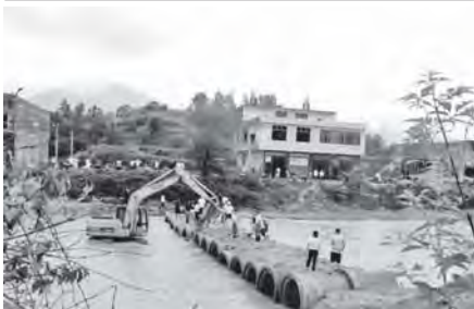
An excavator work to repair a bridge in Huangshaduan Village of Xiushui County, east China's Jiangxi Province, 11 June, 2011. Rain-triggered flood hit the county on Friday. Flood-relief works have been carried out in Xiushui to reduce the economic losses.—XINHUA
