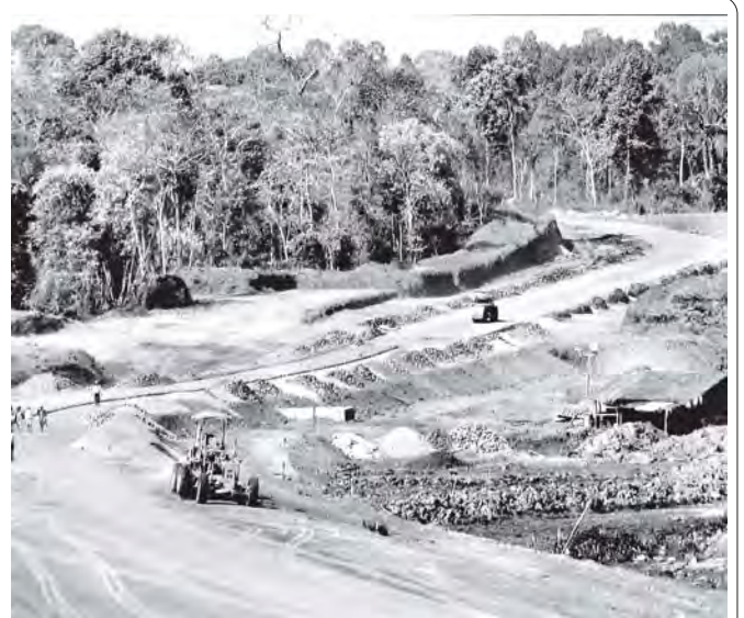
Photo shows a gravel section of Sinkhan-Katha Road Project.
