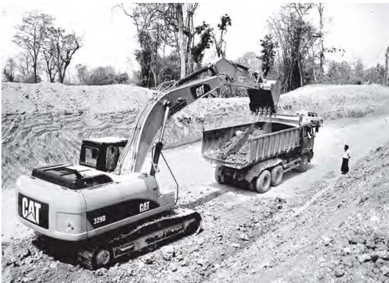
An excavator and a truck at work in Sinkhan-Katha Road Project (65 miles).
