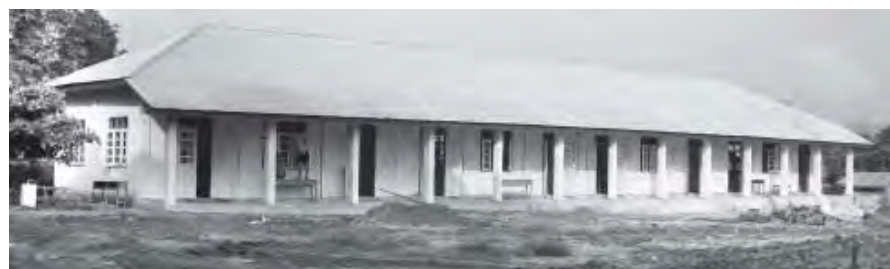
Tahlay Basic Education High School under construction.
