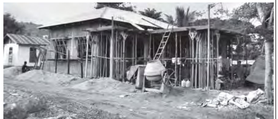
Housing projects in Tahlay nearing completion.
