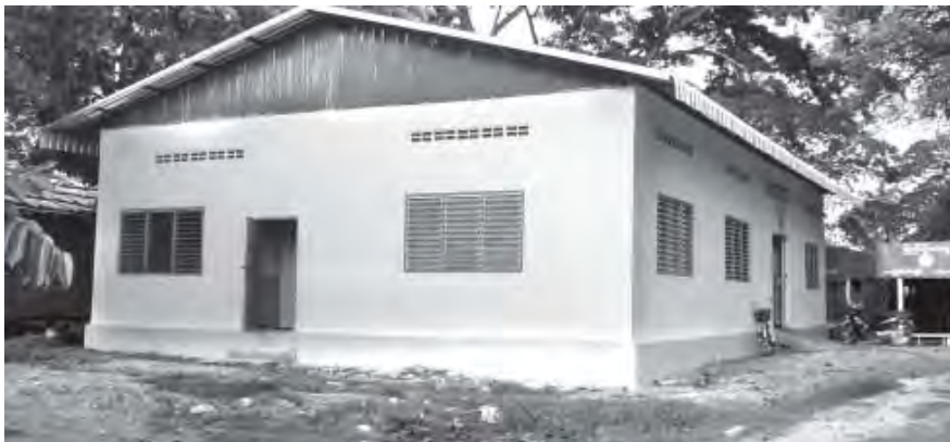
Tahlay General Hospital being built.
