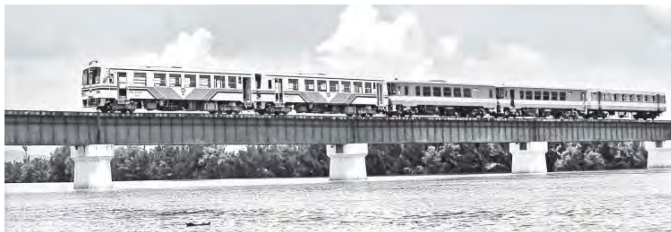
First train running on Dawei-Thayetchaung railroad section of Myeik railroad construction project.—MNA
