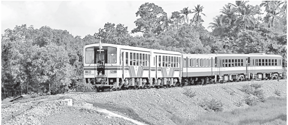
First train running on Dawei-Thayetchaung railroad section of Myeik railroad construction project.—MNA
