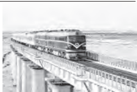
A train runs on a grand bridge of the newly opened "KuiBei Railway", connecting Kuitun to Beitun in northwest China's Xinjiang Uygur Autonomous Region, on 1 June, 2011.
