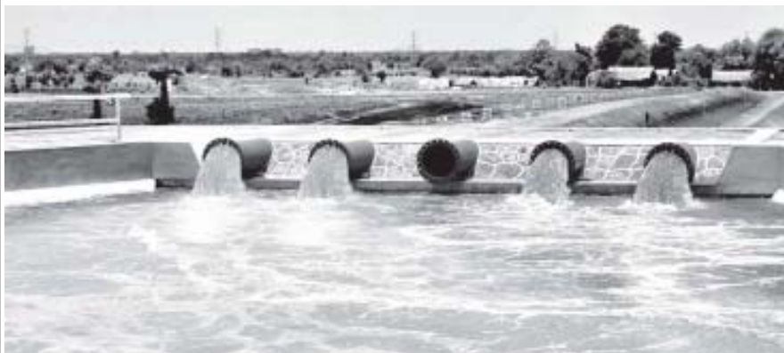
Water is pumped with husk-fired gasifiers through leading channel.
