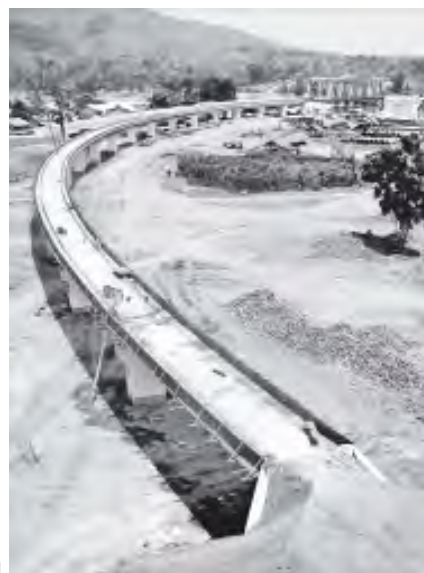
The approach railroad to Ayeyawady Bridge (Sinkhan).
