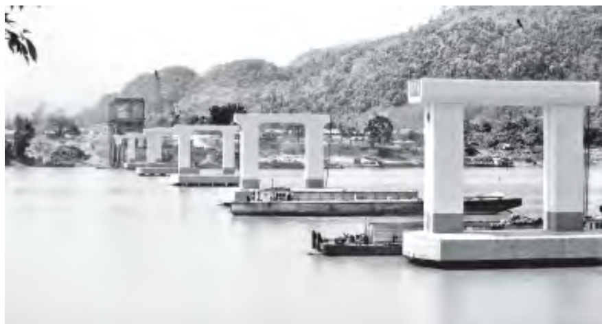
Piers for Ayeyawady Bridge (Sinkhan).
