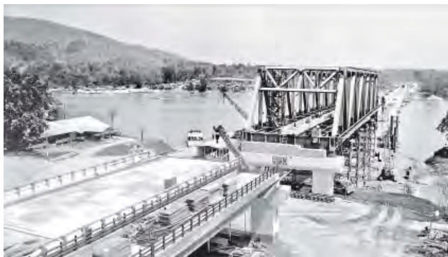
Ayeyawady Bridge (Sinkhan) Project seen with mountain ranges in the background.
