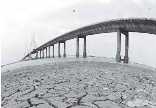
Photo taken on 11 May, 2011, shows the bed full of cracks due to a severe drought under a bridge in the Dongting Lake in Yueyang City, central China's Hunan Province.—XINHUA
