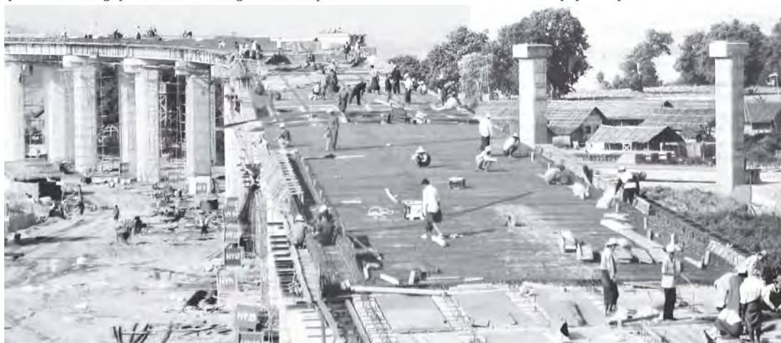
Concrete works being placed on approach road (motor road) of Ayeyawady Bridge (Malun) on Migyaungye bank.
