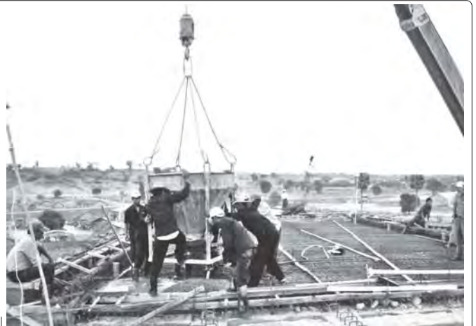
Workers building Ayeyawady Bridge (Malun).
