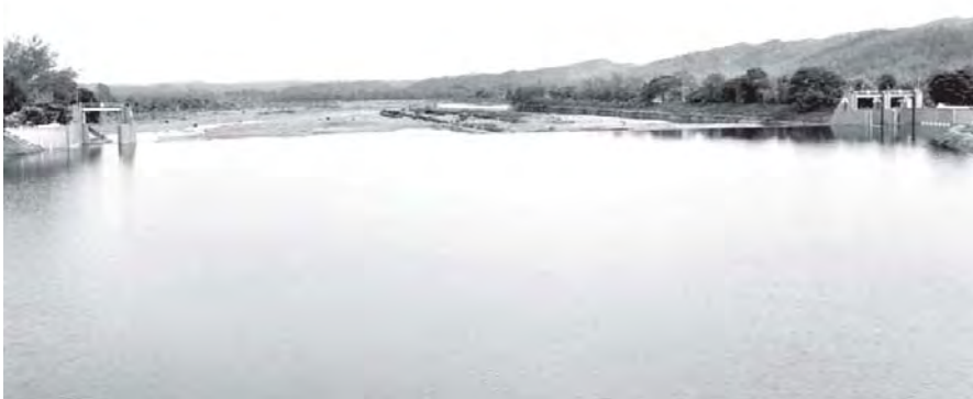
IRRIGATION FACILITY IN MAGWAY REGION: Aingma Diversion Weir was built on Mann Creek near Aingma Village of Minbu Township, Minbu District, Magway Region in 1891. The 580 feet long and 10 feet high concrete facility is supplying water to annual and perennial crops on irrigated areas.
