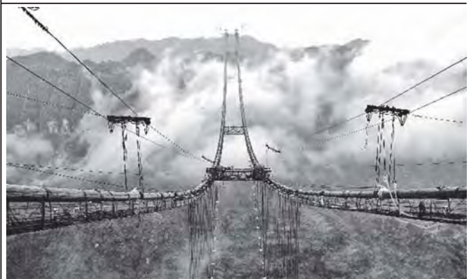
Photo taken on 2 May, 2011 shows the Aizhai suspension bridge under construction in western Hunan Province, central China. The steel truss girder structure has the country's longest suspension bridge main span of 1,176 meters.—XINHUA
