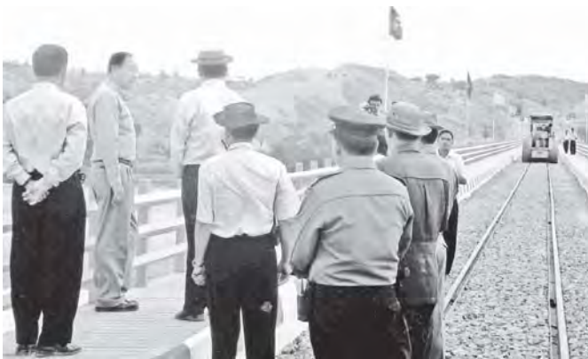
Chief Minister U Phone Maw Shwe inspects Yawchaung Bridge.—MNA
