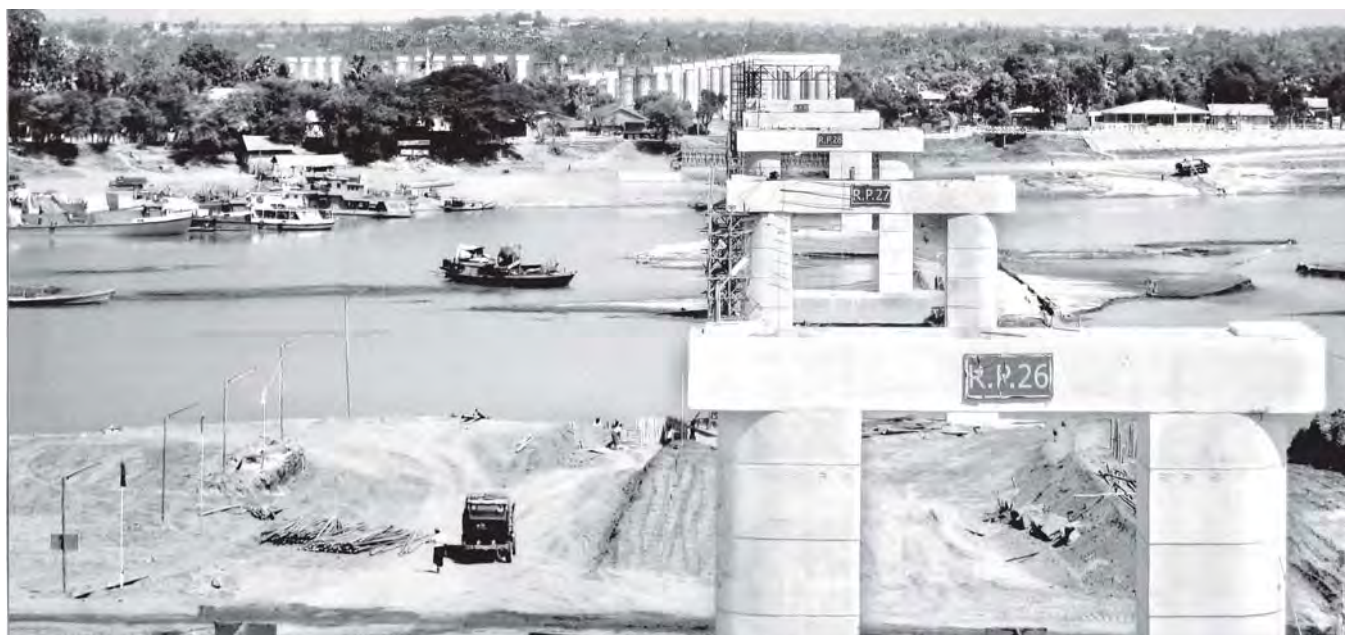
Photo shows sandbank in Ayeyawady River and piers for main structures of Ayeyawady Bridge (Pakokku).
