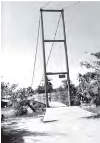
The suspension bridge crossing Bago River.
